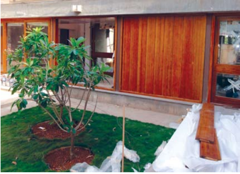
Ritikaa's exterior cladding comes in ready-to-assemble panels which fit tightly together.
