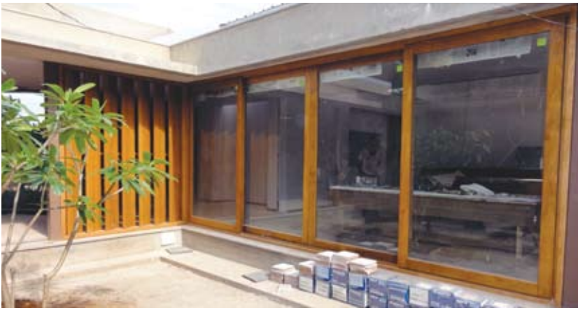
Sliding doors are a particularly attractive option which can provide excellent temperature and sound insulation when closed and maximum airflow when opened.
